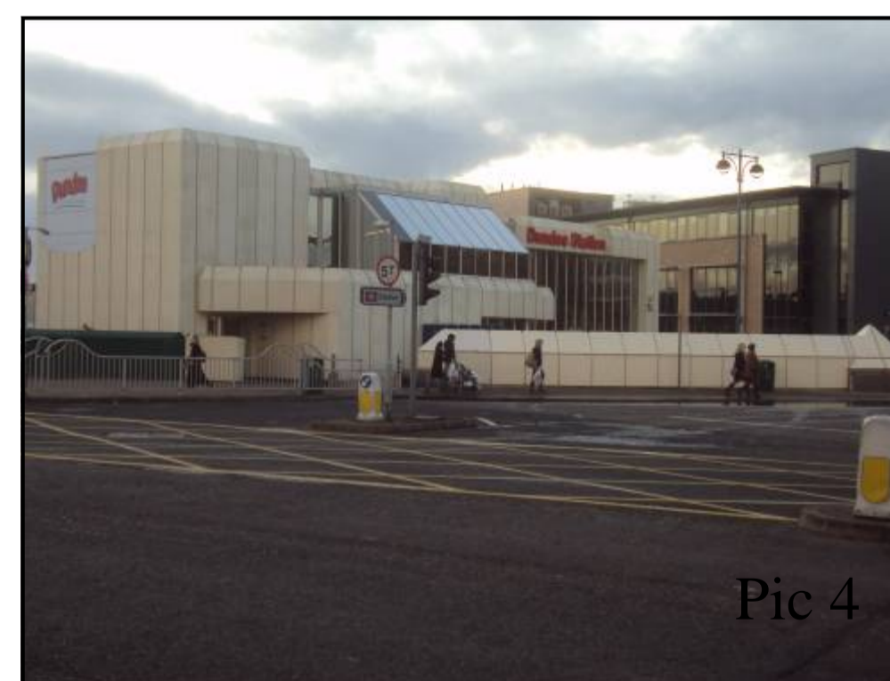
Pic 4 shows the current façade of the rail station. (all pictures that are without a reference have been taken personally.)
