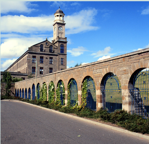
The new development
