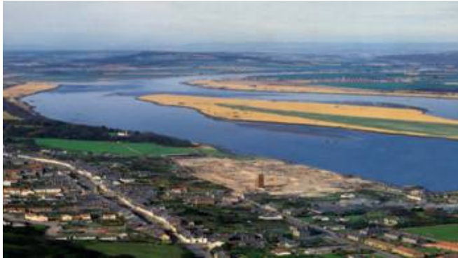
Linoleum factory site after demolition: M. Burgess
